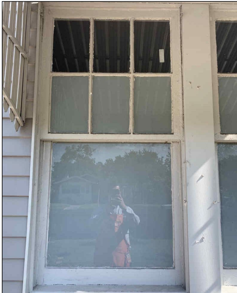
Figure 2: Photograph of historic window to be replaced.
